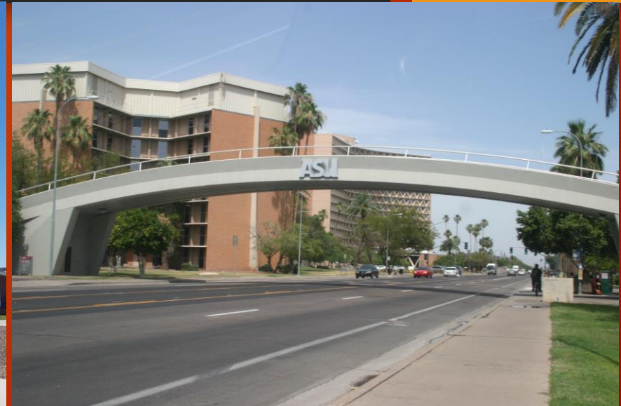
ARIZONA STATE UNIVERSITY PEDESTRIAN BRIDGE [11]
